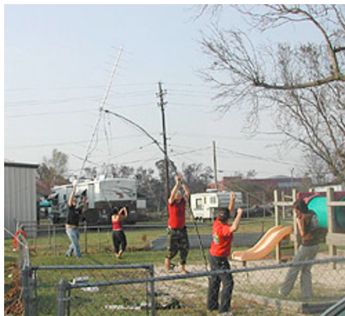
Rhode Islander Matt Hackman, KB1FUP (center), and youth from a local Baptist church erect a VHF Yagi for use in Pensacola, Mississippi. The antenna helped establish a VHF link to Ocean Springs, Mississippi. (Matt Hackman, KB1FUP, photo)
